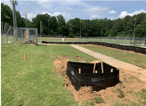
FD- Temporary Fence and Erosion Control
